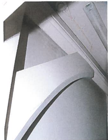
30. 1888 centre roof kingpost and brace adjacent to lift area.J...
