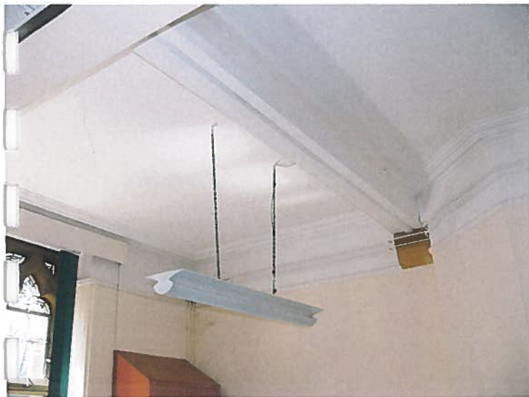
25 1888 west end first floor beam support with 1910 alteration...
